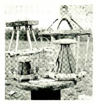
Fig. 21—Two types of insulators used in guy wires of WJZ antenna.
